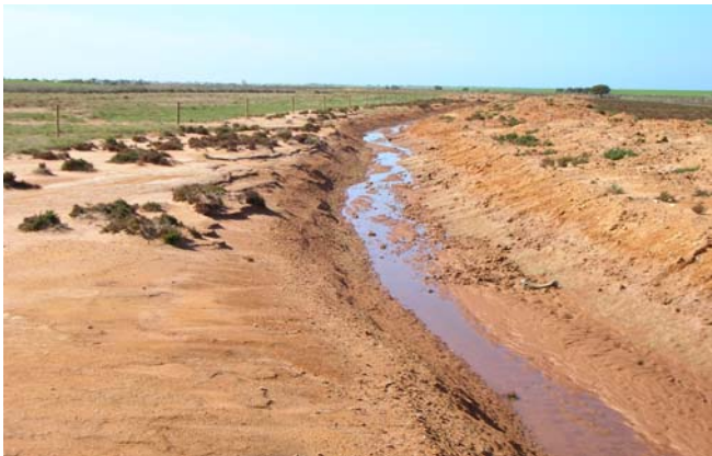
Drainage helps move surface water and groundwater across the low-lying coastal creek flats.
